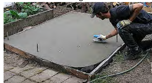
1.2. The finished foundation ready to cure.
