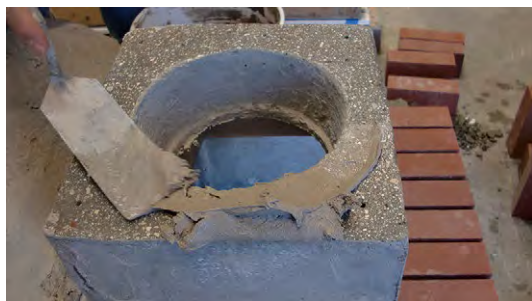
6.4. Apply a bead of refractory mortar.
