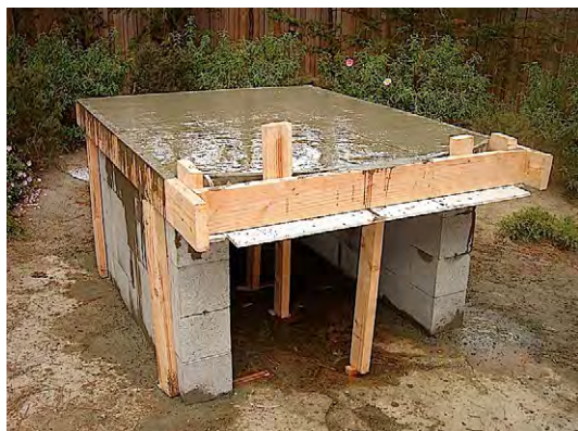
3.5 Structural layer waiting on insulating layer.
