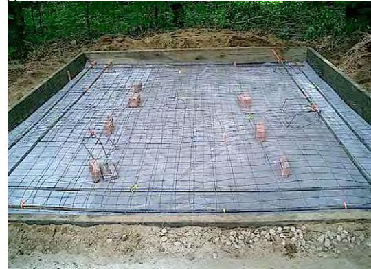
1.1. Framed, lined, with wire mesh and rebar.
