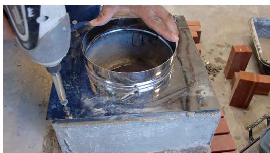
6.5. Screw the anchor plate in place.
