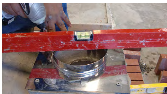
6.6. Check for level.
