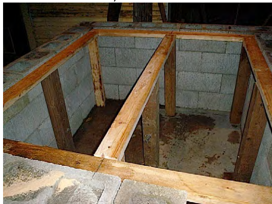
3.1. The form bottom ready for the Hardibacker.
