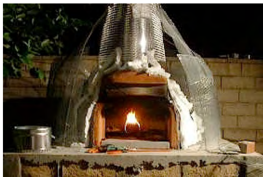
9.1 Rebar and lathe shape the Igloo.
