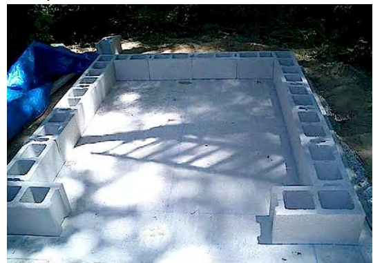
2.1. Carefully lay out the first course of blocks.
